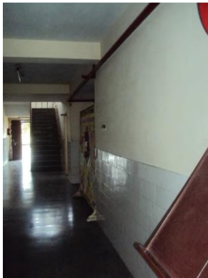
Fig. Emergency Exit
