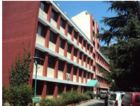
Fig.: 1 Type Of Building
