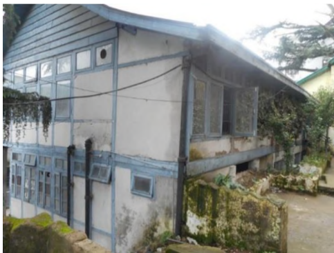
Fig.:3(i)(Sill & Lintel Band)
