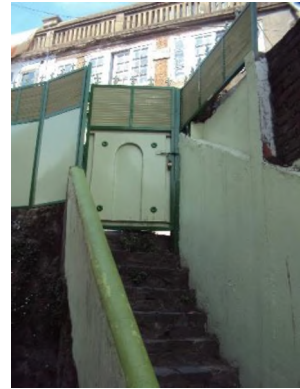
Fig. Emergency Exit
