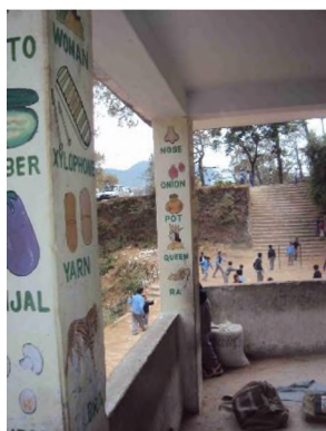
Fig.: RCC Column (no cracks)
