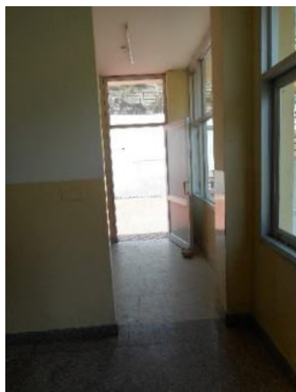
Fig.: Emergency Exit
