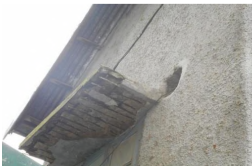
Fig.:Reinforcement Corrosion
