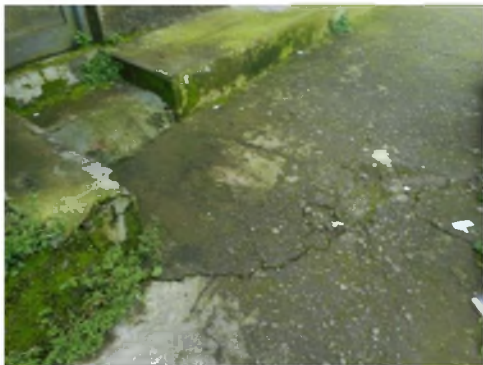
Fig.:Foundation settlement
