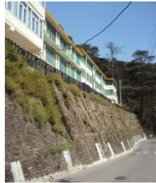
Fig. : Road View
